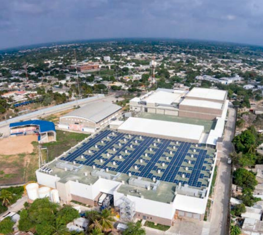
Viva Wajjira, in La Guajira, is one of the five Malls with LEED certification
